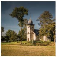
The church was built in 1700 from boulders, with tile roof and tower, Vaulted ceiling is made of unplanned boards and the floor of burned clay slabs. The church has three altars, which were built at different times
